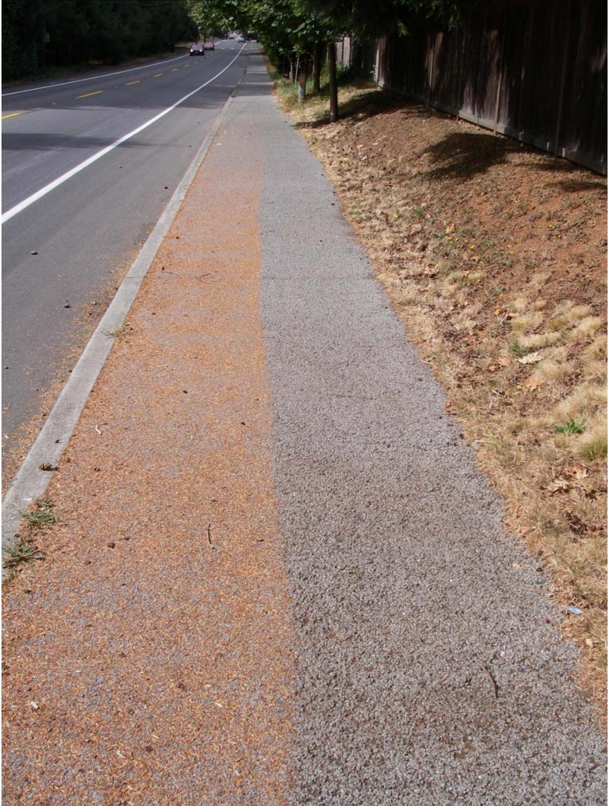
Photo 3. Close up of cleaned and un-cleaned porous sidewalk.
