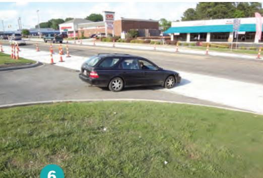
**6** During the curing period, mainline traffic is kept off the RCC pavement, but crossing traffic is allowed at driveways
