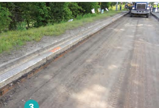
**3** Immediately prior to RCC placement, the pavement is milled an additional eight inches
