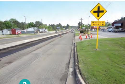
**2** Milling the pavement to lower it two inches below the original gutter elevation
