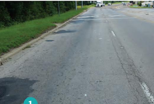
**1** Successive overlays nearly covered the curb while the pavement deteriorated
