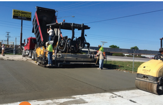
1 RCC process underway.
