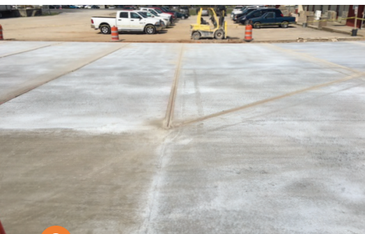
2 RCC concrete successfully joins existing concrete with proper construction joints.
