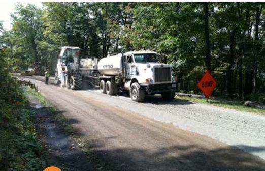
**2** The reclaimer mixes water and cement into the pulverized pavement.
