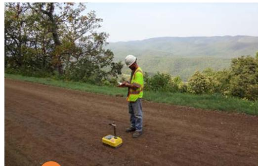
**3** Verifying compaction of the reclaimed base with a nuclear density gauge.
