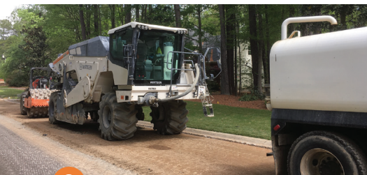
2 FDR process underway
