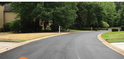
4 Roadway after FDR
