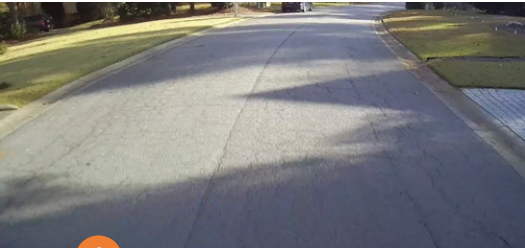
1 Roadway before FDR
