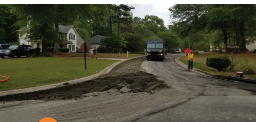
3 Open to local traffic during construction
